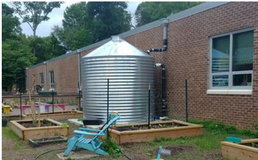
Image 4: Rainfall collection tank and downspout from roof
