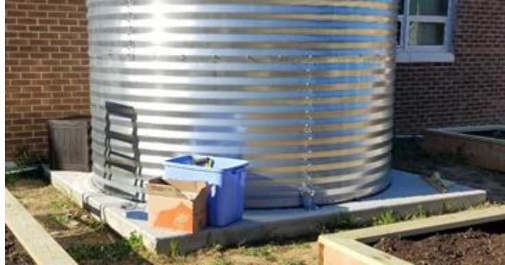
Image 3: Concrete pad supporting rainfall collection tank
